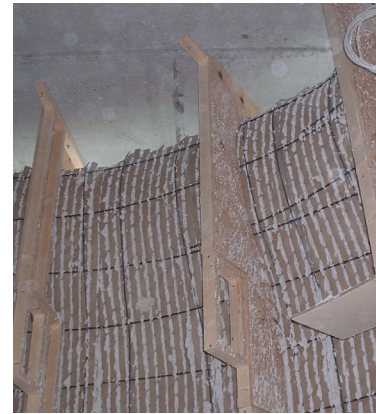
Stucanet base construction
